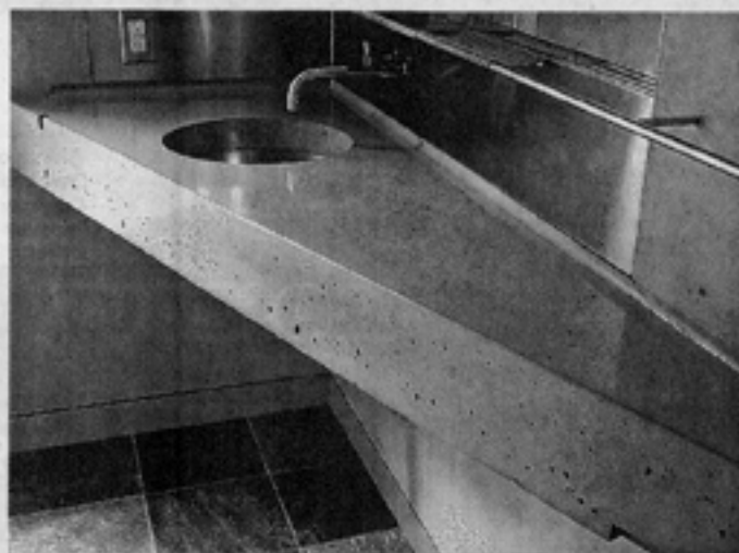
A stylish wedge-shaped concrete counter by Fu-Tung Cheng that also saves space in a small powder room.
