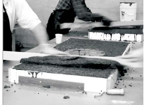
Image 3. Work the screed in a sawing motion
