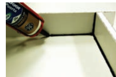
Apply silicone to all corners in the mold.
