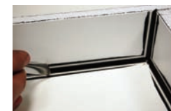
Tooling the silicone with a fillet tool.
