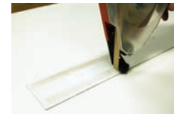
Apply transfer tape to top and bottom of wall liner
