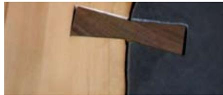
The butterfly joints were made of lpe, an incredibly dense and strong hardwood, to withstand movement between the concrete and wood.
