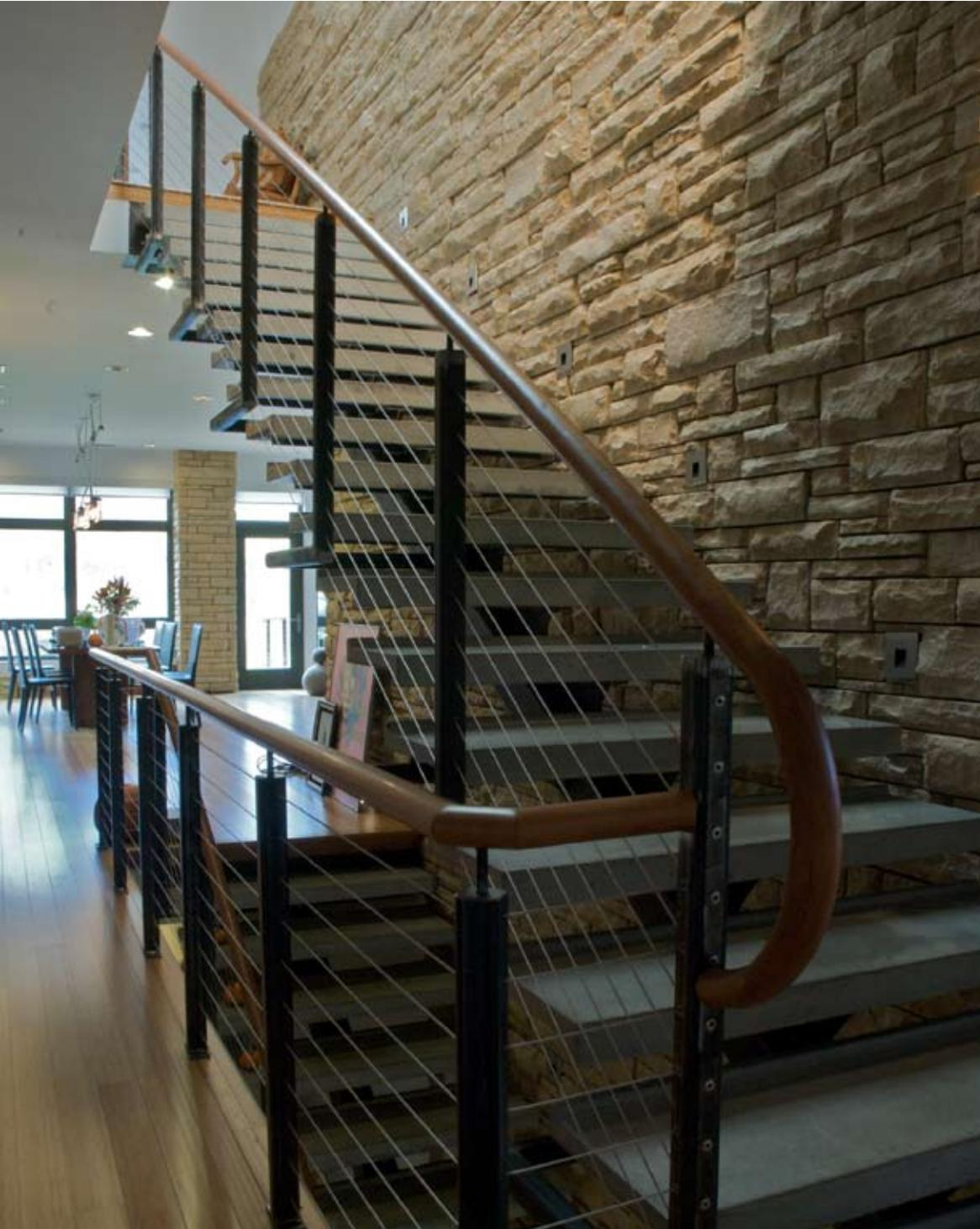
*Left:* To create a gentle curve, the treads shorten incrementally toward the center tread. The wood railing is supported by steel arms mounted to the central spine of the stairs. The stair treads are bolted to the stringer and cantilever out into space, appearing to float.
