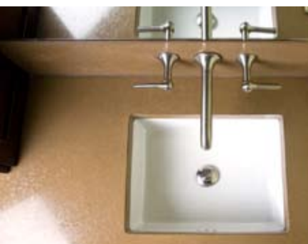
Above: The backsplash was added as the construction progressed because the designer/owner wanted the concrete to look more substantial than it previously would have.
