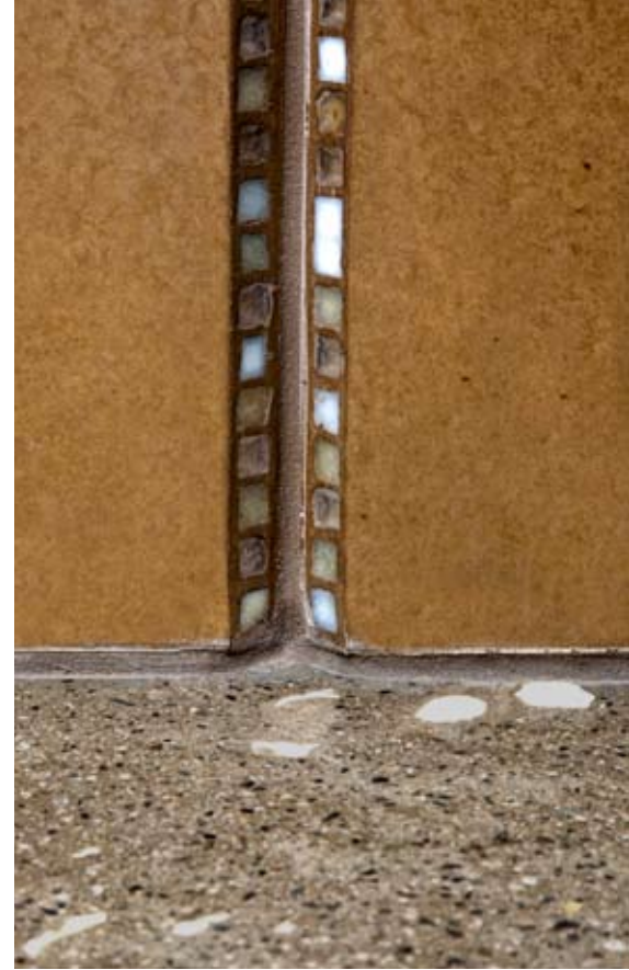
Above: The meticulously embedded tiles in the beveled concrete panel edge add a matching accent to the tiled wall.
