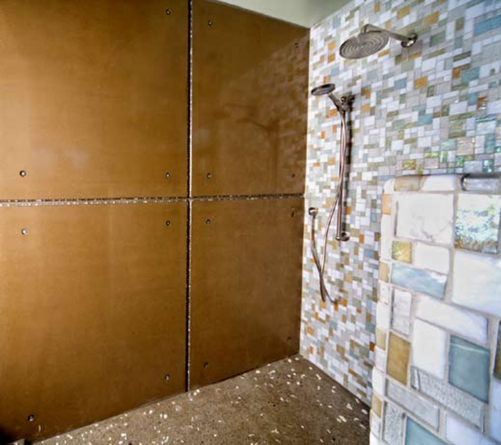
Above: Four foot concrete panels that are only one inch thick are set like tile on this shower wall. The shower pan was poured in place using sea shells as a decorative aggregate and then polished like terrazzo.
