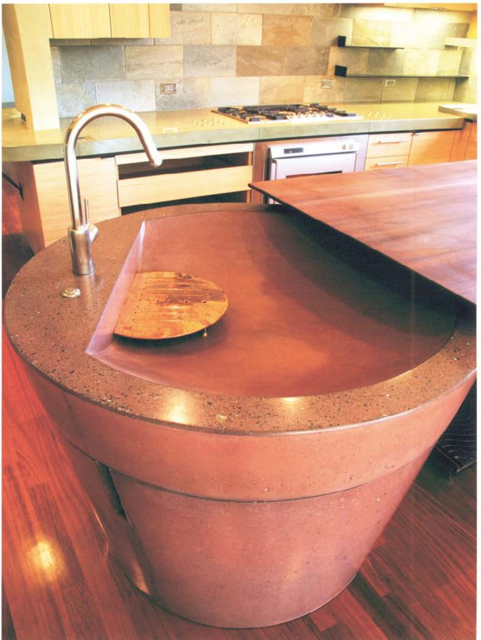
Above: The integral concrete sink includes a custom copper strainer ■ Opposite page (top): The entry canopy is made of steel and delicately interwoven twigs that lace just beneath the glass surface
