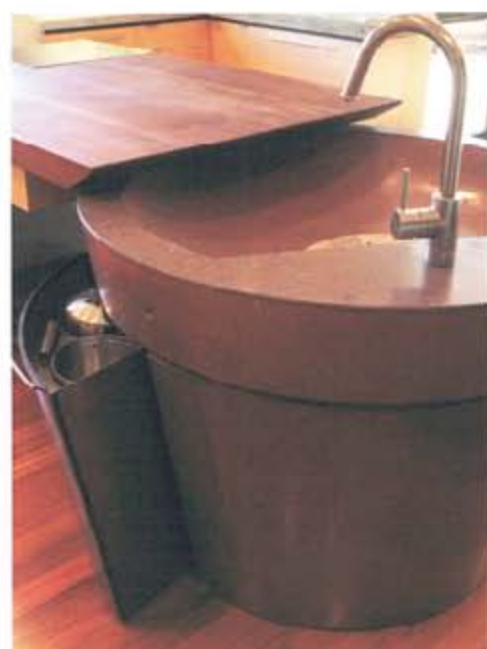
Above: The island counter is made with mahogany and Geocrete concrete ■ Bottom: An ammonite shell has been imbedded into the countertop ■ Right (top): Attention to detail is seen in the roof structure and the interesting geometric patterning of the window panes ■ (middle and bottom): The compost and trash bins are built into a pull-out drawer in the conical sink support
