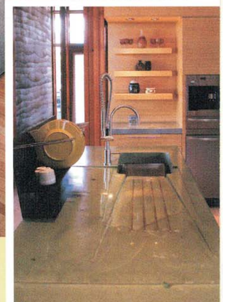
RIGHT: Brass bars inlaid directly into the concrete countertop form a drain board that slopes into the sink.
