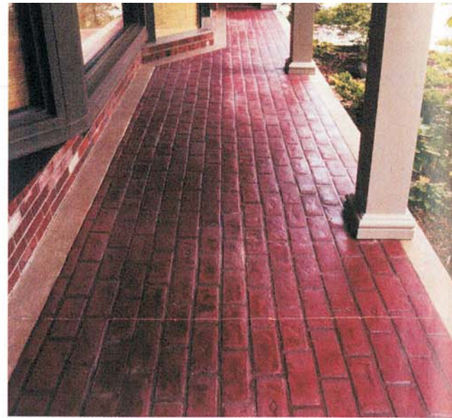
At this Lafayette, Ind., home, decorative concrete was cut to replicate bricks for the walkway. Photo by L.M. Scofield Company 2005
