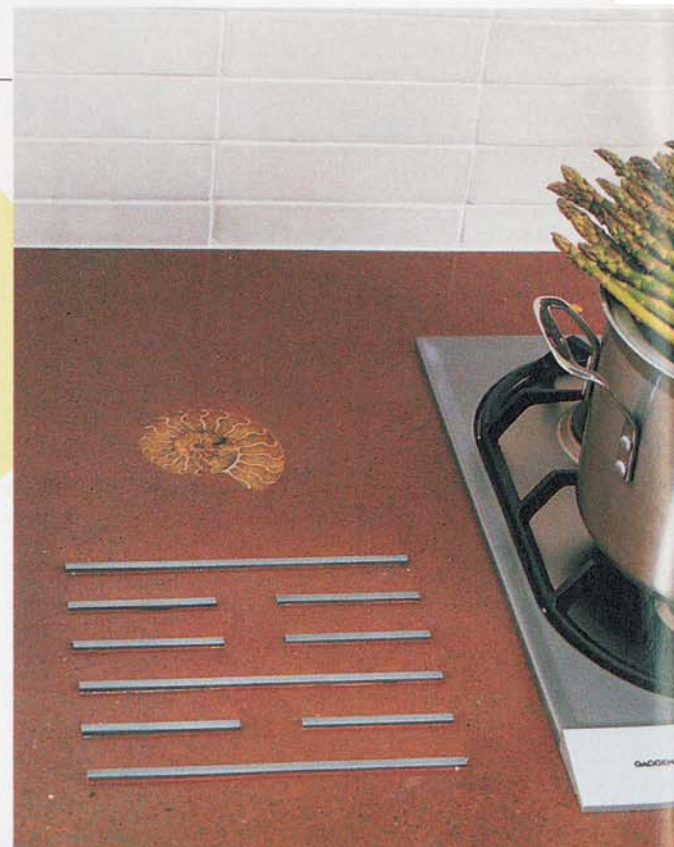
BELOW: In the hands of an expert like Cheng, concrete becomes an artist's canvas. Inlaid steel rods make a resting pad for hot pots; a fossil adds unusual beauty.
