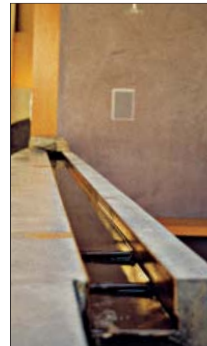
Creative concrete designers are constantly looking for new objects to inset, new colors and textures to cast and new applications for the material. Here a circulating waterfall is cast into the top of a 22-ft.-long interior wall.
