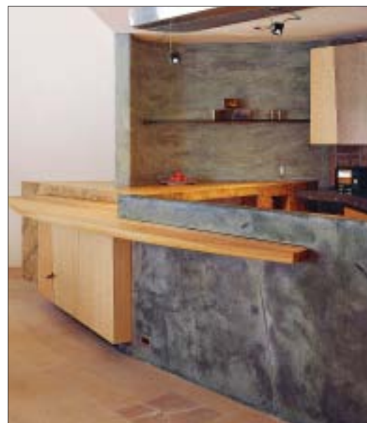
Like horizontal castings, vertical projects can be cast in place or cast off-site and installed. This divider wall was cast off-site and installed with the cabinets and counters it is integrated into. If you look closely, you can see a small seam in the middle of the wall, running at a slight angle. The angle makes the seam less noticeable and less susceptible to directional stress.
