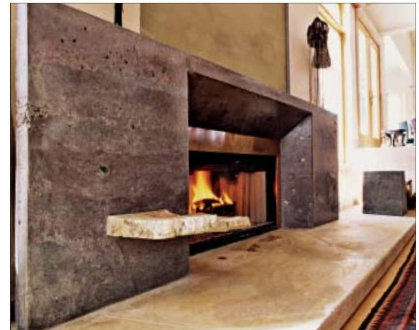
The fireplace is a natural area to shape with concrete. You can use it to cast a hearth, mantel or surround — or all three. If you choose to make adjoining parts from concrete, incorporating complementary differences will make the design more interesting. For example, in the fireplace above, the hearth and surround feature different pigments and finishing techniques. The hearth has a smooth, ground finish typical of a countertop or floor, whereas the surround is less polished — voids and other irregularities are left unfilled to increase visual interest.
