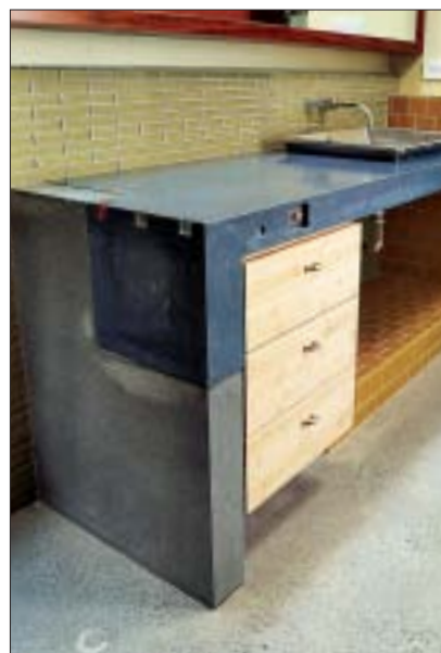
This concrete vanity was cast in two interlocking parts. Although interesting and beautiful, it is not for beginners. Like any other medium, concrete requires experience and skill to yield pleasing results. Try starting with smaller casting and finishing projects (see "Cast Away," May/June 2003, p. 46) and work your way up to more ambitious undertakings.
