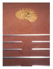
It's also a very functional material. You can't cut drain boards into Corian or Formica, and you can't cut them easily into granite. A drain board is a sculpted area that drains water from your countertop into your sink, the way the Rubbermaid plastic piece that goes under the average dish rack does. With concrete, you don't have to set a plastic drain board on your countertop. The drain board is built in. It's ground in the concrete so that it becomes a functional sculpture.
